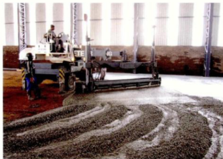
The Somero laser screed machine is part of CLF's large equipment line
