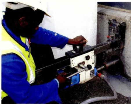
Core drilling leaves clean entry and exit holes – making subsequent sealing easy and neat
