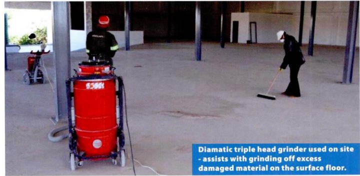
The BMG-435 Diamatic triple head grinder used on site by a contractor.
