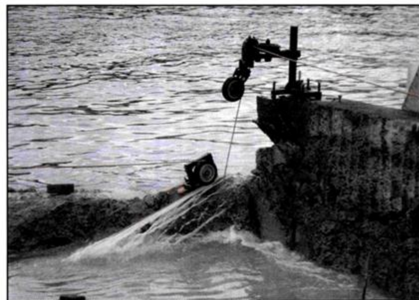
Widening the entrance at the Simonstown Stillwater Harbour.
